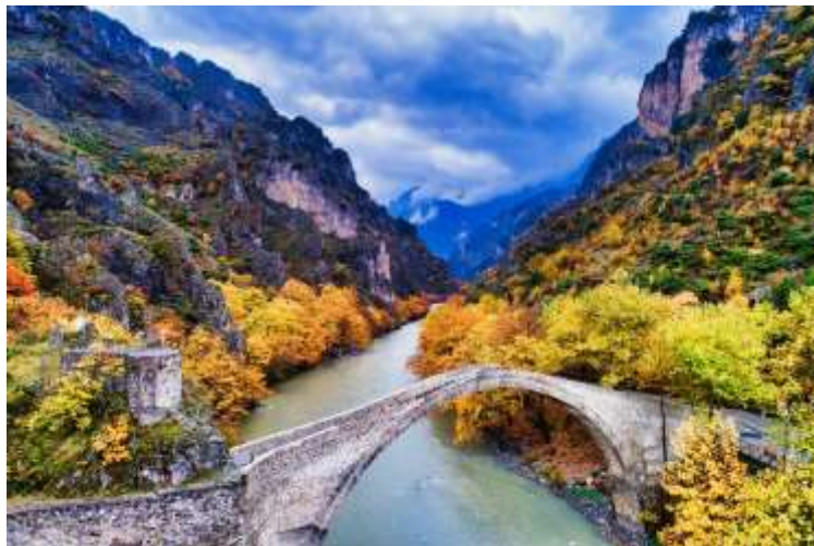
Noutsos stone bridge
